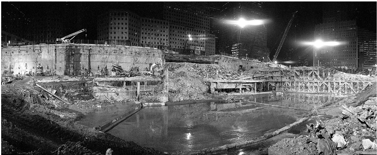
Figure 1. The WTC bathtub prior to rebuilding of the 1/9 subway lines (seen middle ground).
